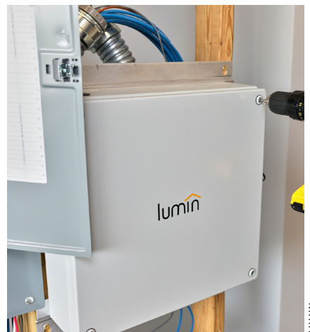
Smart breaker boxes, like the hardware-agnostic Lumin Smart Panel shown here, turn standard panels into smart panels by providing comprehensive energy control and extending whole-home backup.
